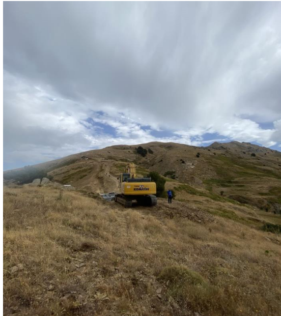
Figure 6-4: Turbine Area - Access Road
