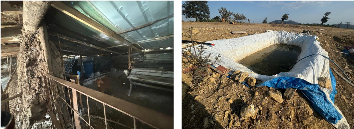
Figure 5-1: Photos of affected house
